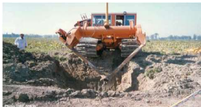
Figure 3. V-plough trenchless drainage machine
